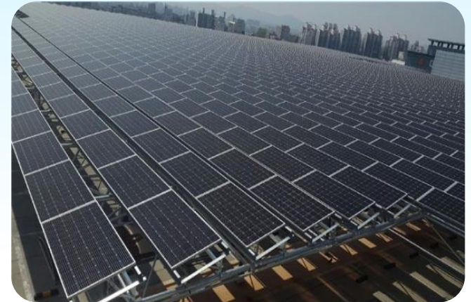
< Rooftop solar panels at express bus terminal
