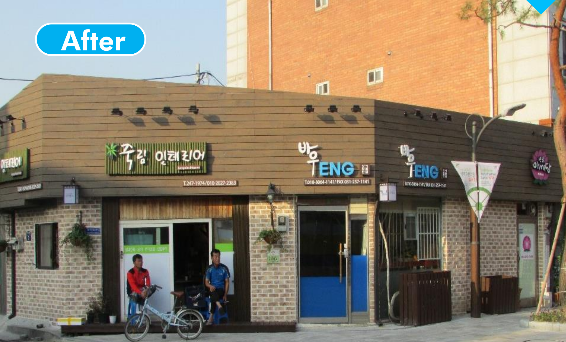
Renovation of Old Sign Boards
